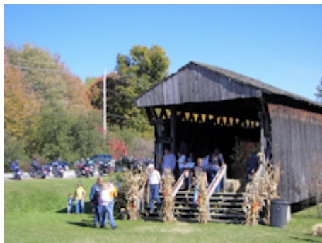
Graham Road Bridge
