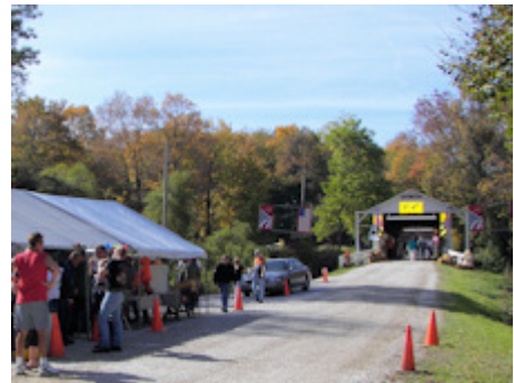
Root Road Bridge
